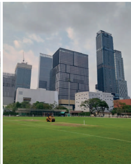
▲ Heavy roller gets to work at the RBSC Polo Ground
